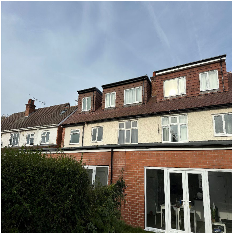
Rear elevation, no. 74 to the left
